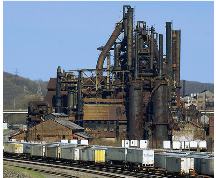
An abandoned steel plant in Bethlehem, Pennsylvania (demolished in 2007)
