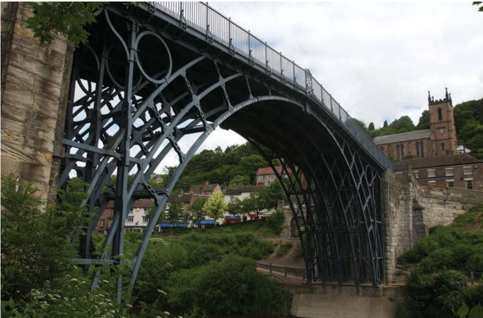
Figure 12.3 Ironbridge, England. The world's first bridge made entirely of cast iron was constructed in the late eighteenth century near Coalbrookdale, England, reflecting the resources, technology, and available skills in this area at the time. © John Robertson/Alamy.
